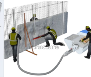
INJECTING THE WALLS
