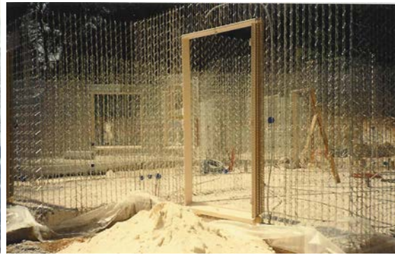
INJECTING THE WALLS
