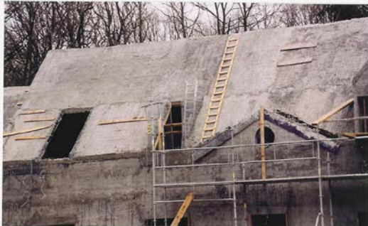
INJECTING THE CONCRETE ROOF
